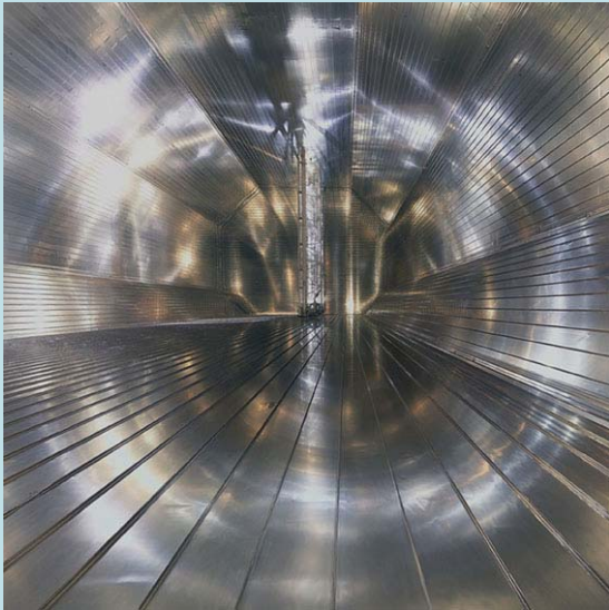
Figure 2: To insulate the tanker CS1 insulation technology was employed for the first time. This allows reduction of the composition of the insulating layers and their thickness to such an extent that the capacity of the tanker was increased by 8,000 m 3 .
