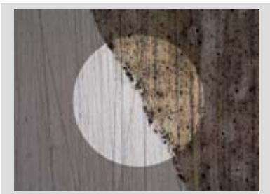
Under the microscope the region protected by the plasma layer exhibits no sign of corrosion even after direct exposure to the salt spray test for 96 hours
