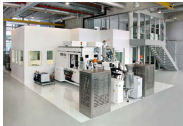
Production in Gira's clean room. Additional filters and laminar flow modules over the handling and mould area of the externally connected injection moulding machine ensure an unchanging quality of air during the entire production process.
